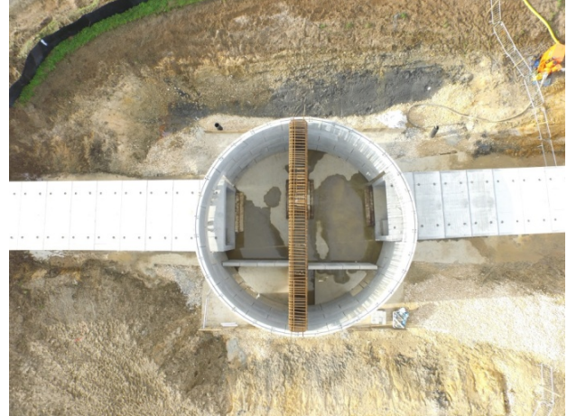
Steelwork fixed to central dividing wall
