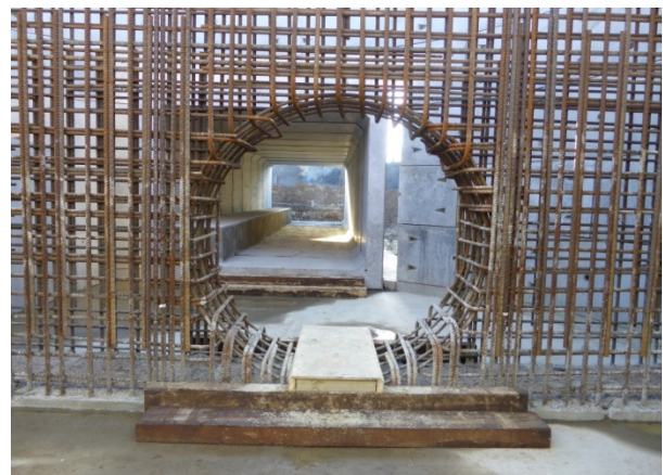
Internal view of control structure
