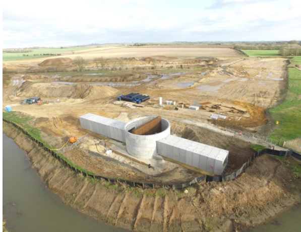
Arial view of control structure
